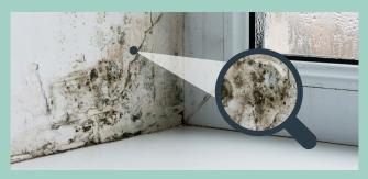
When warm air meets cold surfaces, it turns to water droplets. This is common around windows, in corners, and behind furniture.
