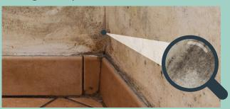
Groundwater rising up through floors and walls, usually due to damp proofing issues.
